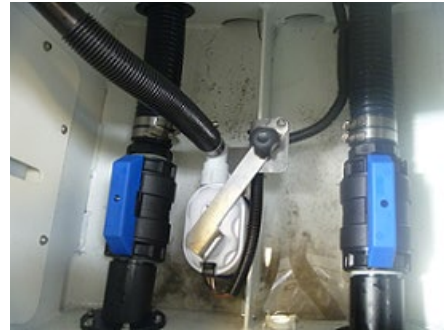
Inside Pod Centre Access Hatch
